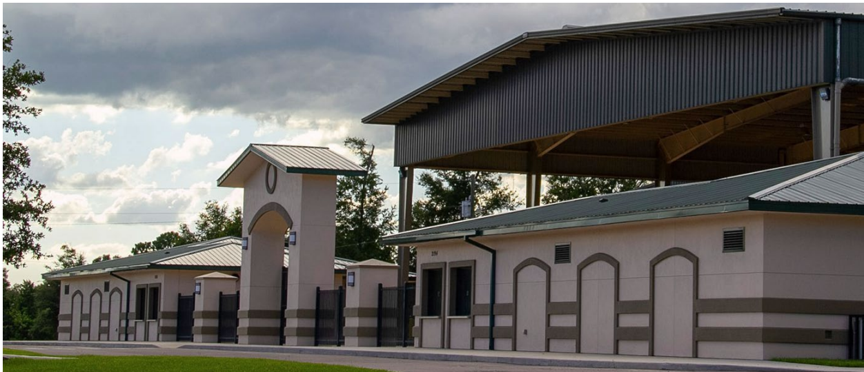
Figure 3: SELP Main Entrance
