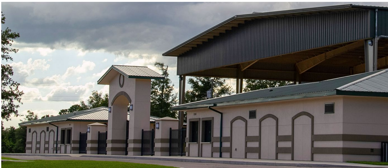
Figure 3: SELP Main Entrance
